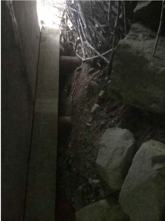
Right Bank Abutment when facing downstream
